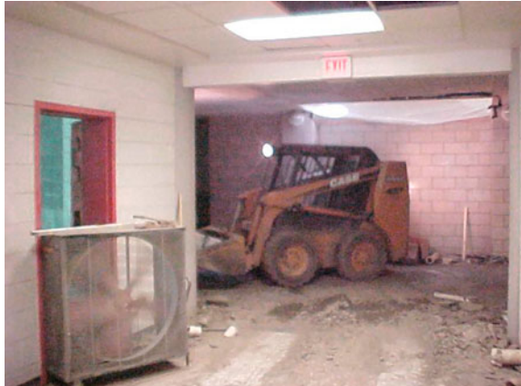
Fig. 15 Interior of Middle School showing Bobcat loader removing existing concrete slab flooring (2006)
