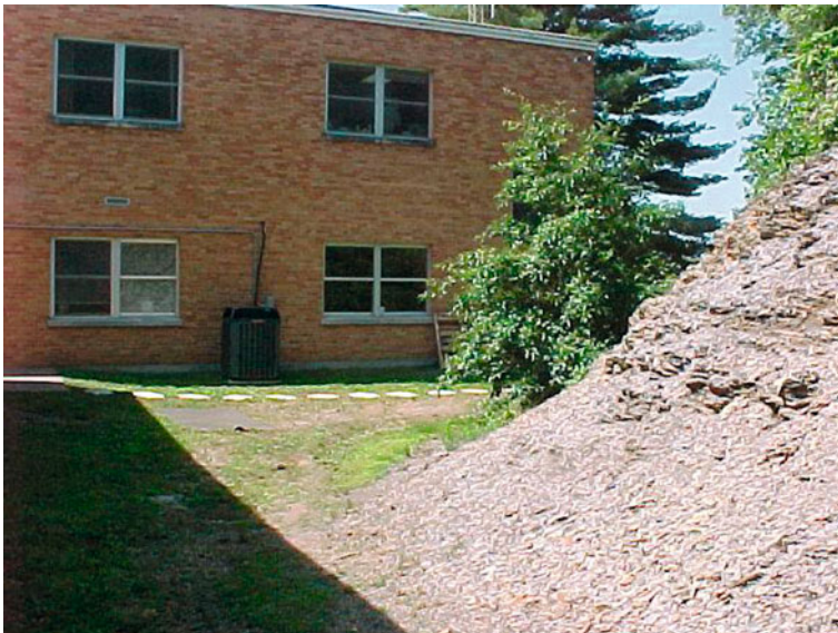
Fig. 26 Exterior of the Marcum and Wallace Hospital office wing and an adjacent outcrop of the Cleveland Member of the Chattanooga (Ohio) Shale. Note the absence of cracks or offsets in the load bearing walls and exterior brickwork of rooms with heaved floor slabs
