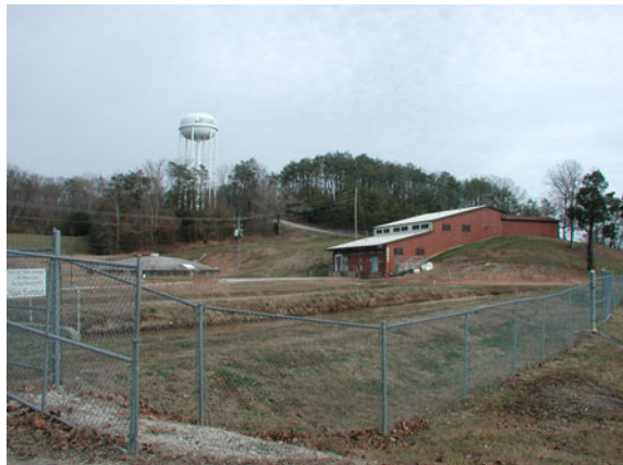
Fig. 29 Clay City (Beech Fork) Water Treatment Plant
