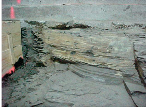
Fig. 18 Cleats with sulphate precipitate in Shale beneath Middle School; note new concrete columns
