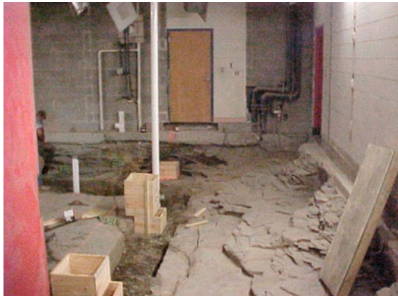
Fig. 16 Shale beneath School and new trench construction for column footers, new and old sewer PVC pipe, cleats with the sulphate mineral
