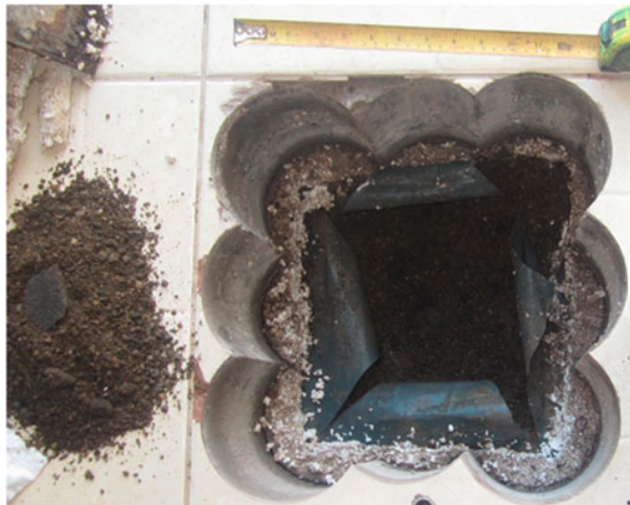
Fig. 5 Blinding sand is carefully removed and a small sample taken immediately after the membrane has been cut and bent back
